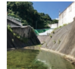
Flood control reservoir
