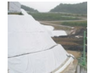
Seepage control work
