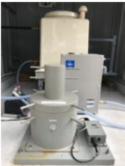
Continuous measurement system for groundwater radioactivity concentration
