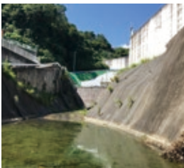
Flood control reservoir
