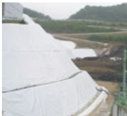
Seepage control work
