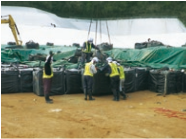
Upper section : Landfill of cement solidified waste and non-cement solidified waste
