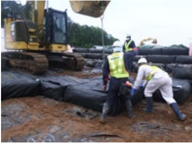
Lower section : Landfill of non-cement solidified waste
